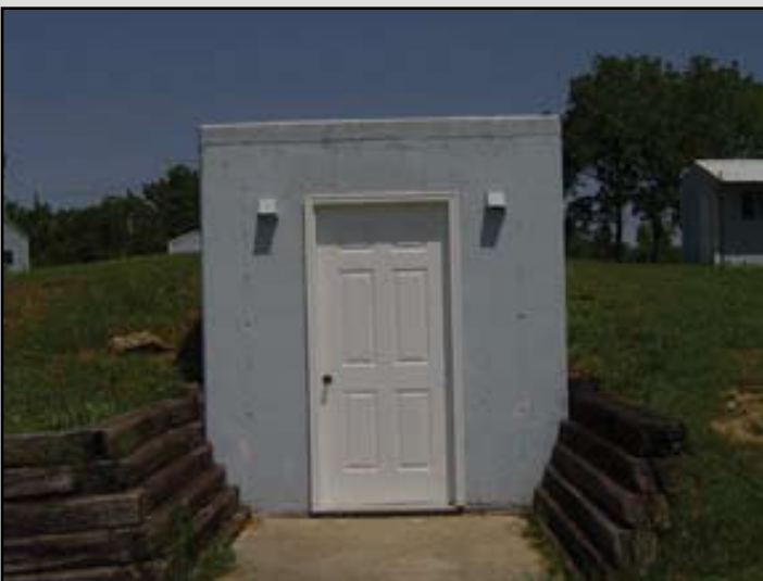
Storm Shelter (concrete, carpeted, ventilated)
